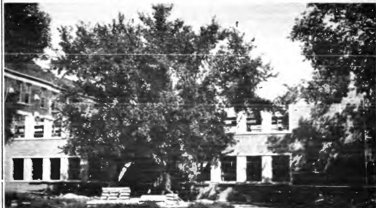
Another addition to the NDAC campus, the agriculture engineering building, will be ready next spring. The building is located Northwest of the main Engineering building.
