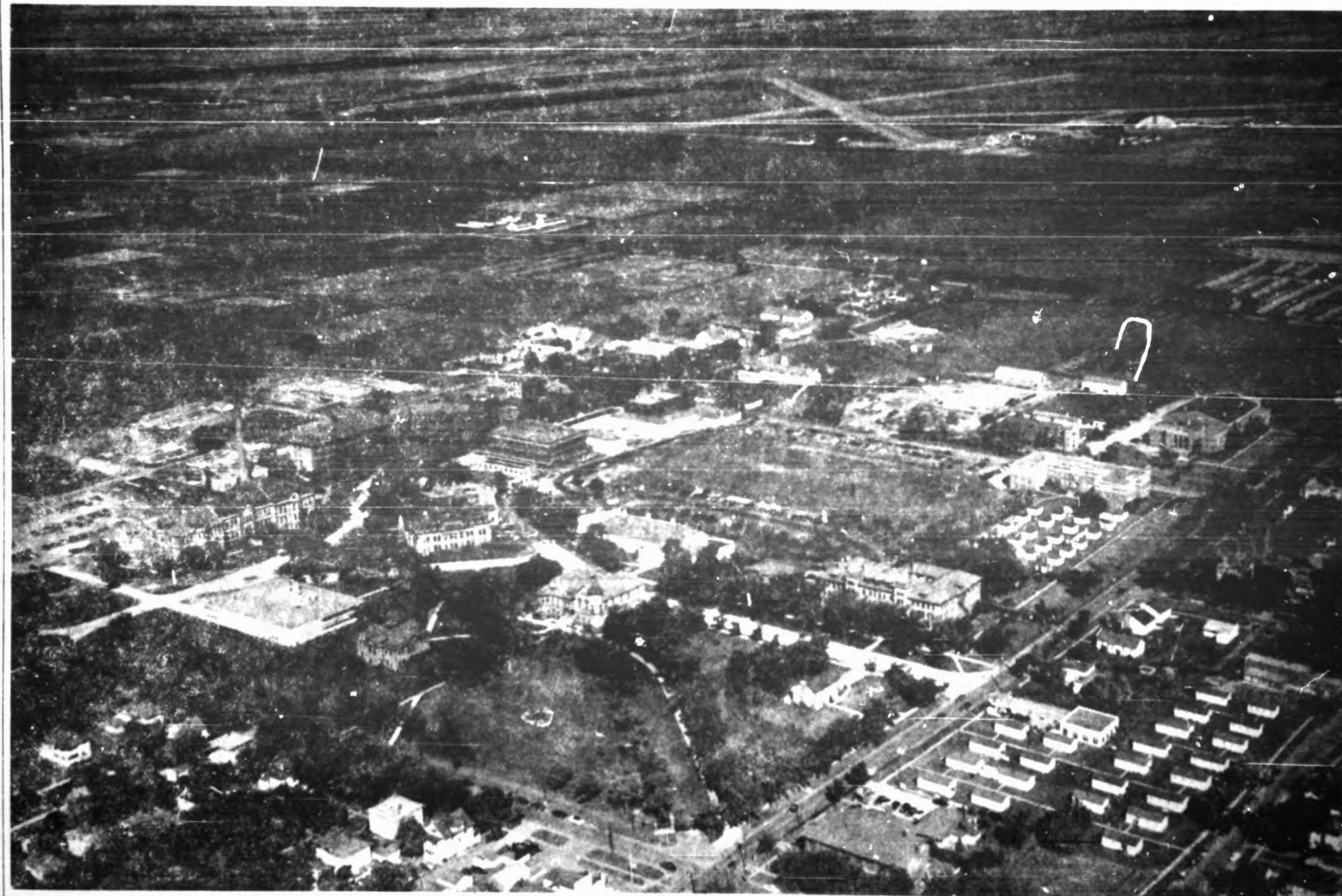
The photograph above, by Merle Nott, shows the NDAC campus from the air during the late summer 1951. The new agricultural Engineering building is located just south of the Chemistry building. West of the Field House the foundation and some of the steel structures of the new Engineering building can be seen. The old Dairy barn will be torn down. On the west end of old Dacotah Field, facing east, the Student Union will be built. The new Home Economics building is also planned for the site of Dacotah Field, just west of the Men's Dorm. Lying northwest of the main campus is the Poultry Research Center.
