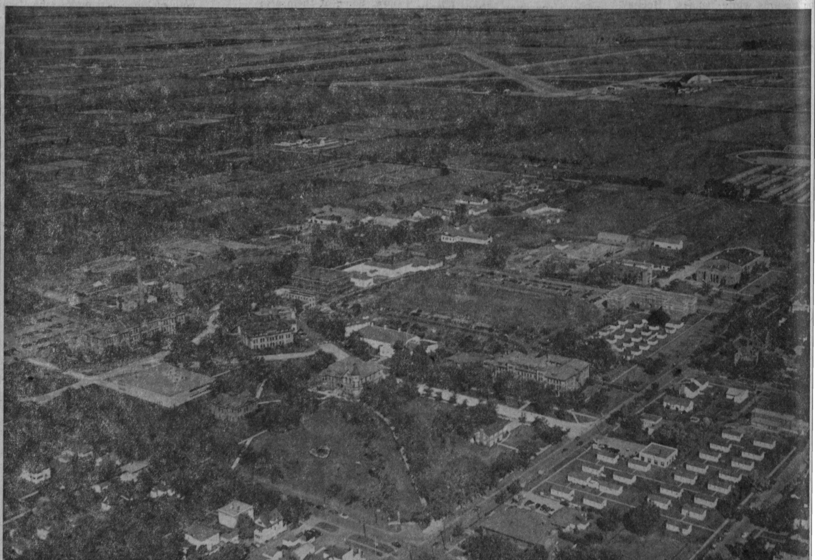
The photograph above, by Merle Nott, shows the NDAC campus from the air during the late summer 1951. The new agricultural engineering building is located just south of the Chemistry building. West of the Field House the foundation and some of the steel structures of the new Engineering building can be seen. The old Dairy barn will be torn down. On the west end of old Dacotah Field, facing east, the Student Union will be built. The new Home Economics building is also planned for the site of Dacotah Field, just west of the Men's Dorm. Lying northwest of the main campus is the Poultry Research Center.
