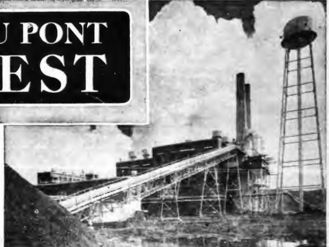
This powerhouse for a nylon plant at Martinsville, Va., was designed by Du Pont engineers. It houses two 135,000 lb. hr. boilers and two 7,500 KW extraction turbine generators.
