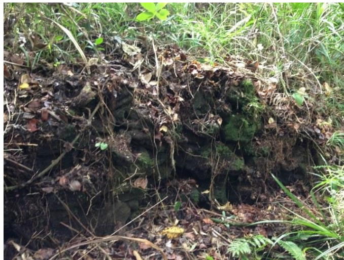
Figure 5. Rock wall from 2014 survey of Mt. Lata trail.
