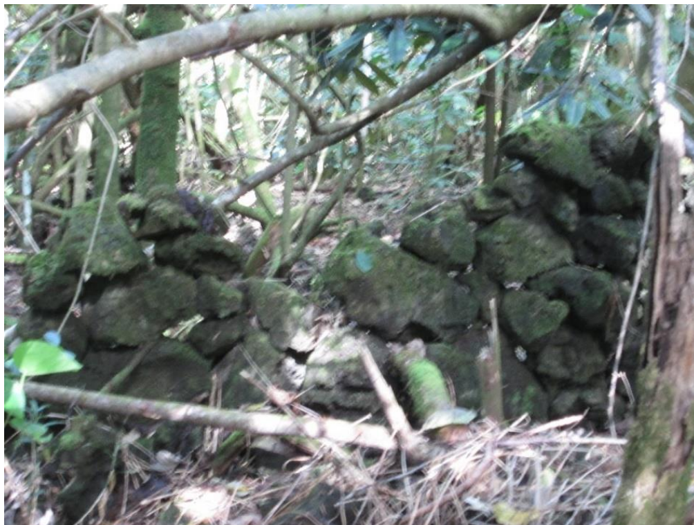
Figure 67. Closer look at the wall.
