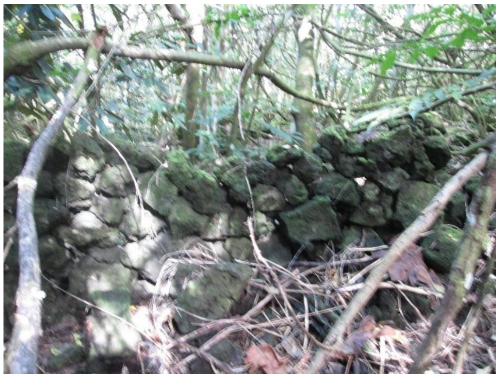
Figure 68. Closer look at the wall.
