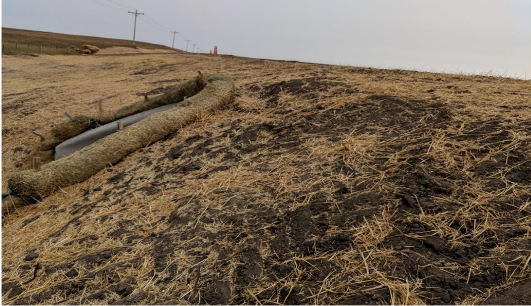
Figure 12: Pipe Work and backfilling at HWY 1804, North Dakota
