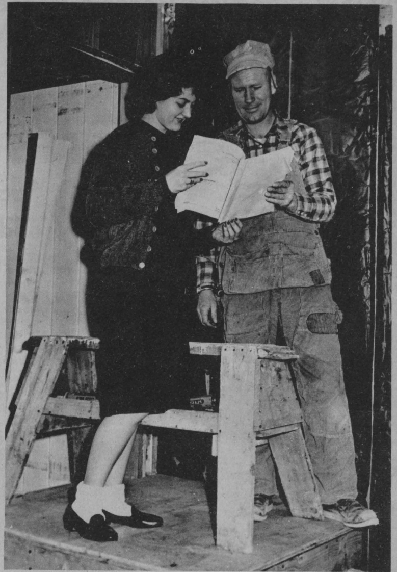
BETTE MOEN is going over the house plans with one of the construction men.
