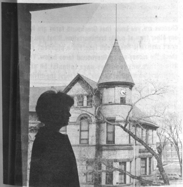
VIEW OF THE OLD FROM THE NEW. Joan Virden looks out a third floor window in the new women's residence, Burgum Hall, which frames the Administration Building, the university's first structure. Workman have completed plastering the building and are installing clothes closets and finishing work.
