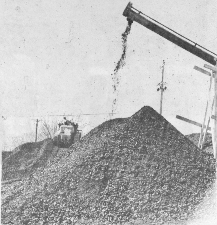
NO, THIS IS NOT a coal mining 312 lab. Twenty boxcars of coal are being dumped behind Minard. The mountain of coal will remain there until the power house is completed.
