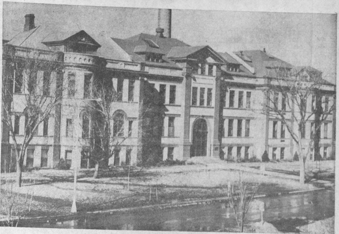
ARTS AND SCIENCE HEADQUARTERS, Minard Hall, is one of the largest classroom buildings on campus. Yet arts and science classes spill over into several other buildings.
