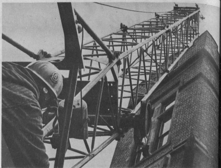
PORTABLE CRANE hoists tower sections to the roof of Ladd Hall
