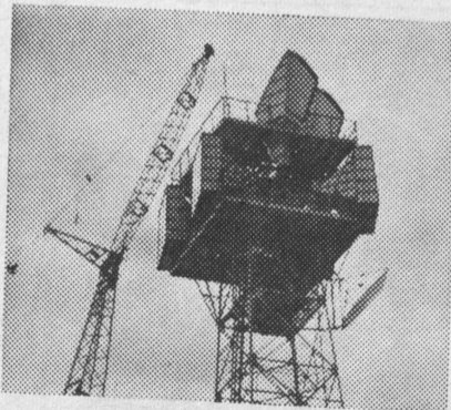
and over the land . . . to provide the world's finest communications
