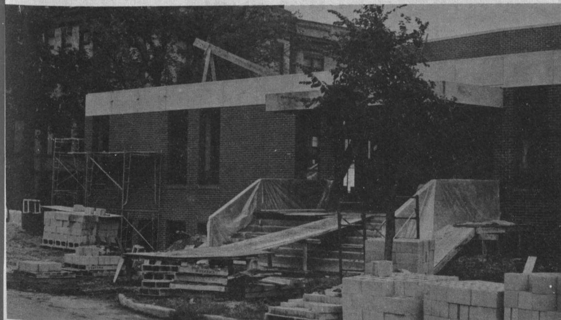
Construction on new Little Country Theatre scheduled for April completion.
