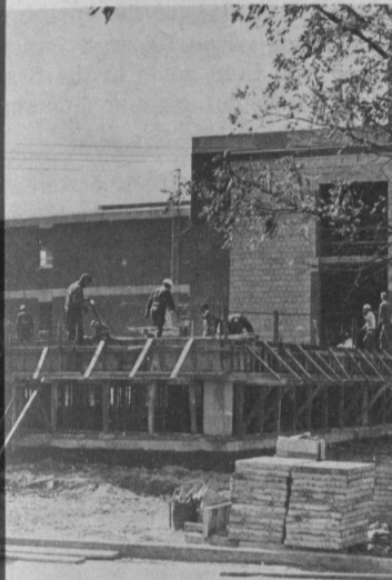
Work proceeds on Phase II of Biological Science Building.
