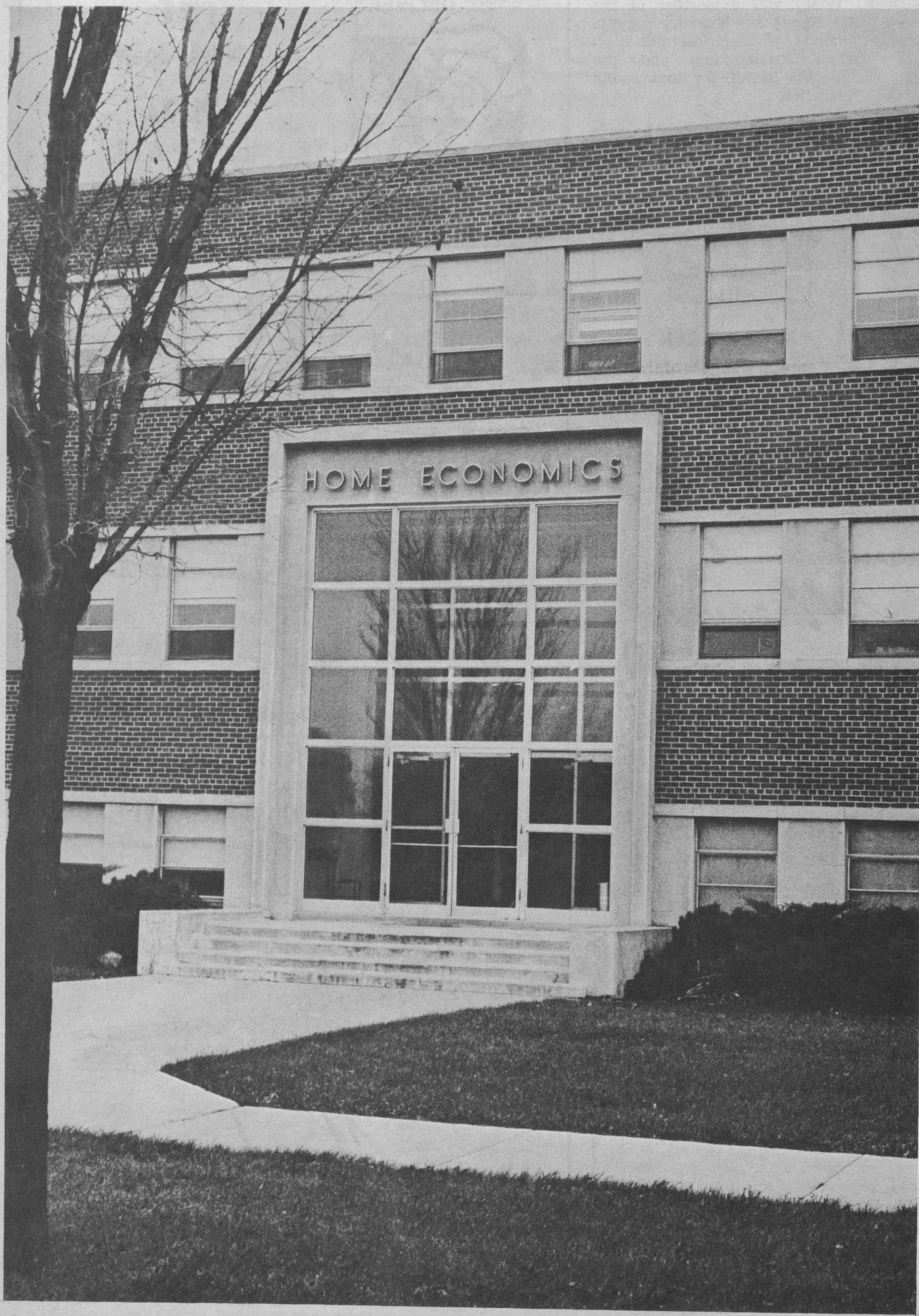
Home Economics Building faces Mall from north.
