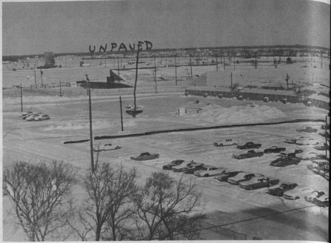
The Reed-Johnson parking lot. The area in the foreground is paved; the area in the background is not. (Photo by Casper)
