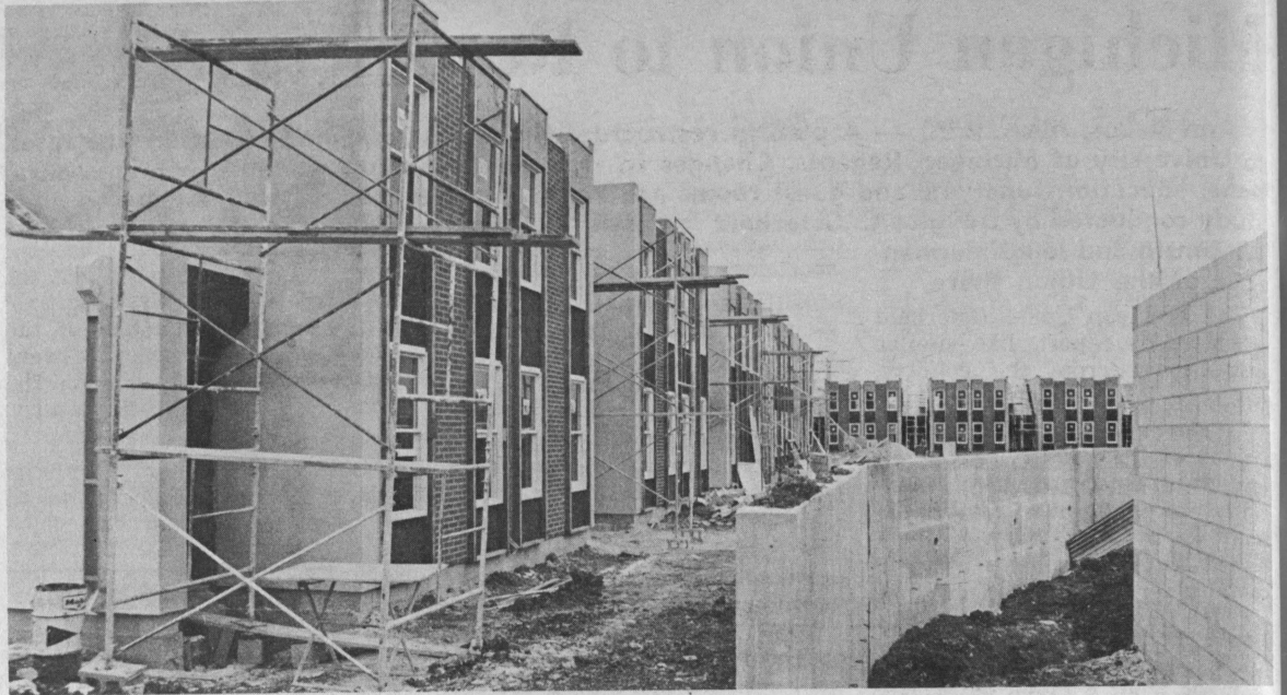
Construction proceeds smoothly on the improved married student housing.
