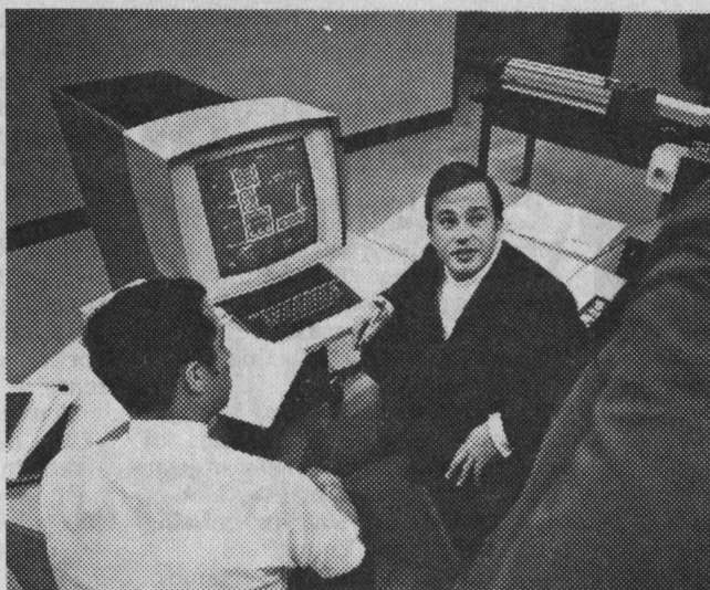
Doug Taylor, B.S. Electronics Engineering '67, is already a senior associate engineer working in large-scale circuit technology. Aided by computer design, Doug is one of a five-man team designing integrated circuits that will go into IBM computers in the 1970's.
