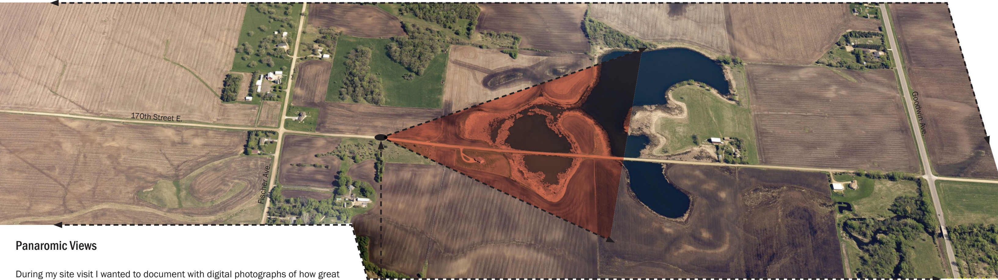
Site Aerial Photo Looking North
