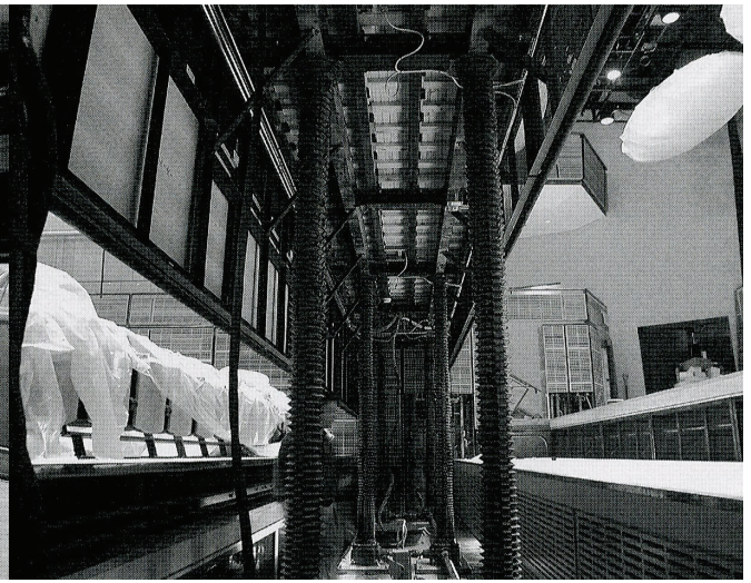
1.14 | Platform lift (for raising and lowering stage/floor)
