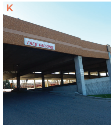
Figure 98 | W Facing SW Empty Parking Garage
