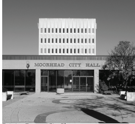
Existing Entry at City Plaza
