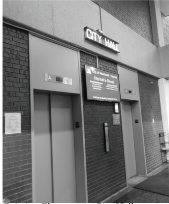
Existing Elevators to City Hall
