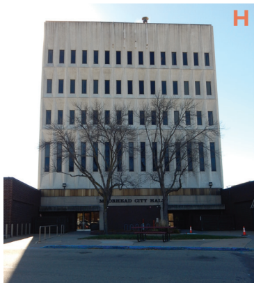
Figure 94 | N Facing S City Hall Entrance
