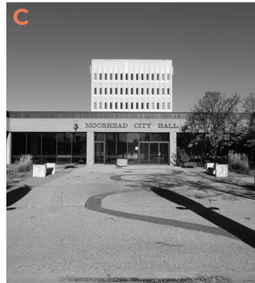
Figure 88 | S Facing N View of City Hall
