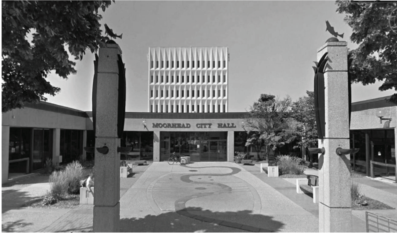
Existing Civic Plaza Center Avenue
