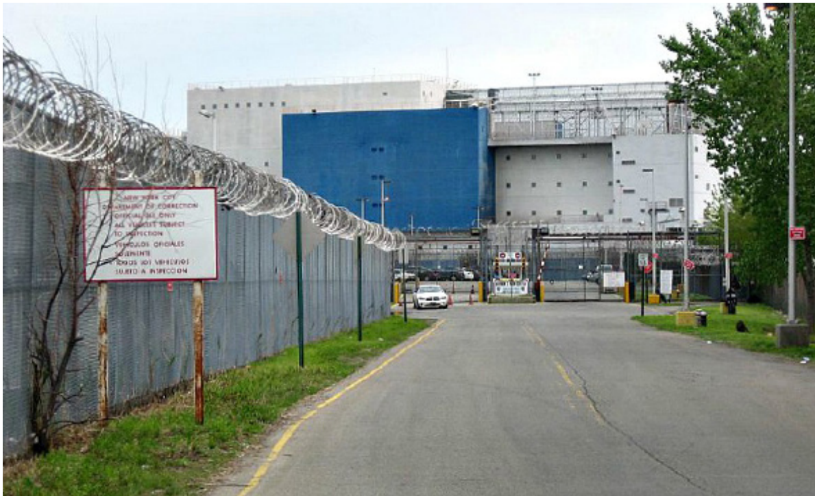
FIGURE 28 | Parking Lot and Main Entrance to the Barge
