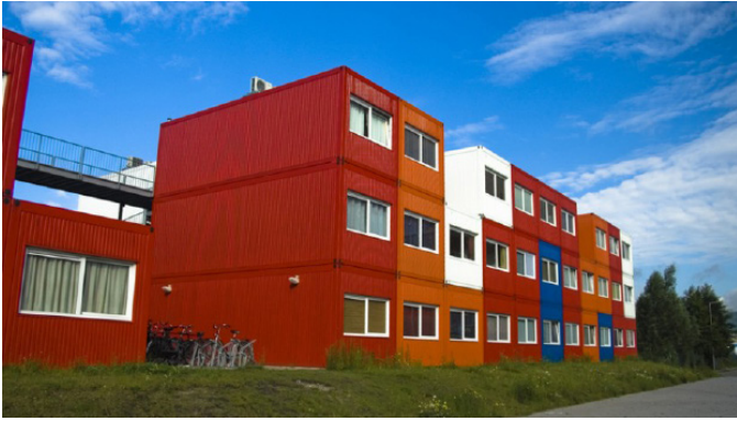
FIGURE 22 | Temporary Container Units - ndsm.nl
