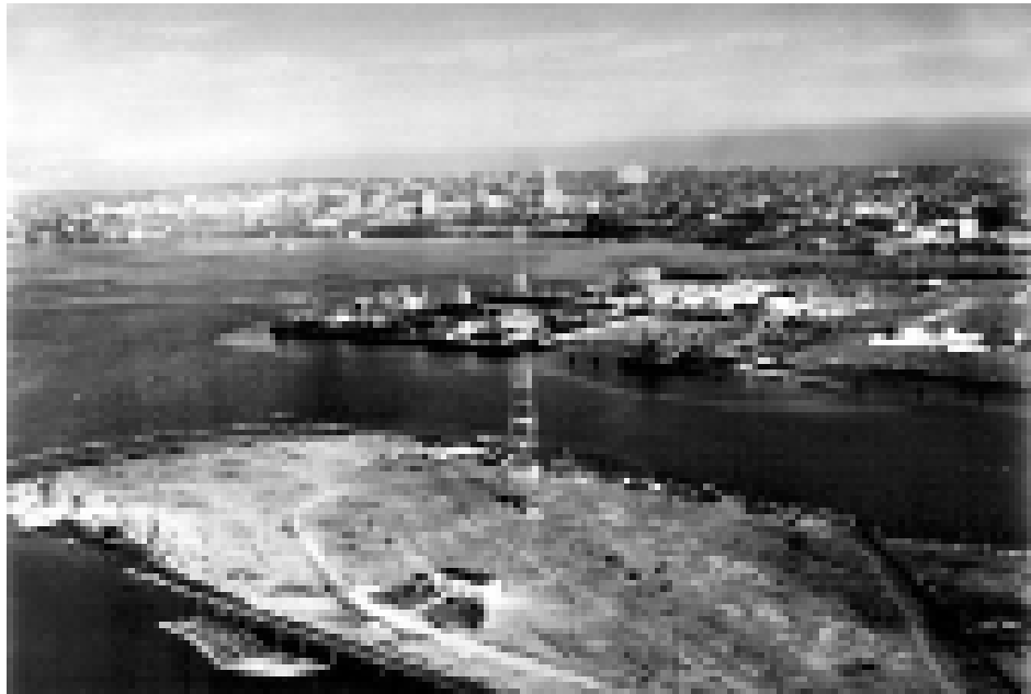
FIGURE 3 | Aerial Views of the KOMO KJR Transmitter on Harbor Island 1936.
