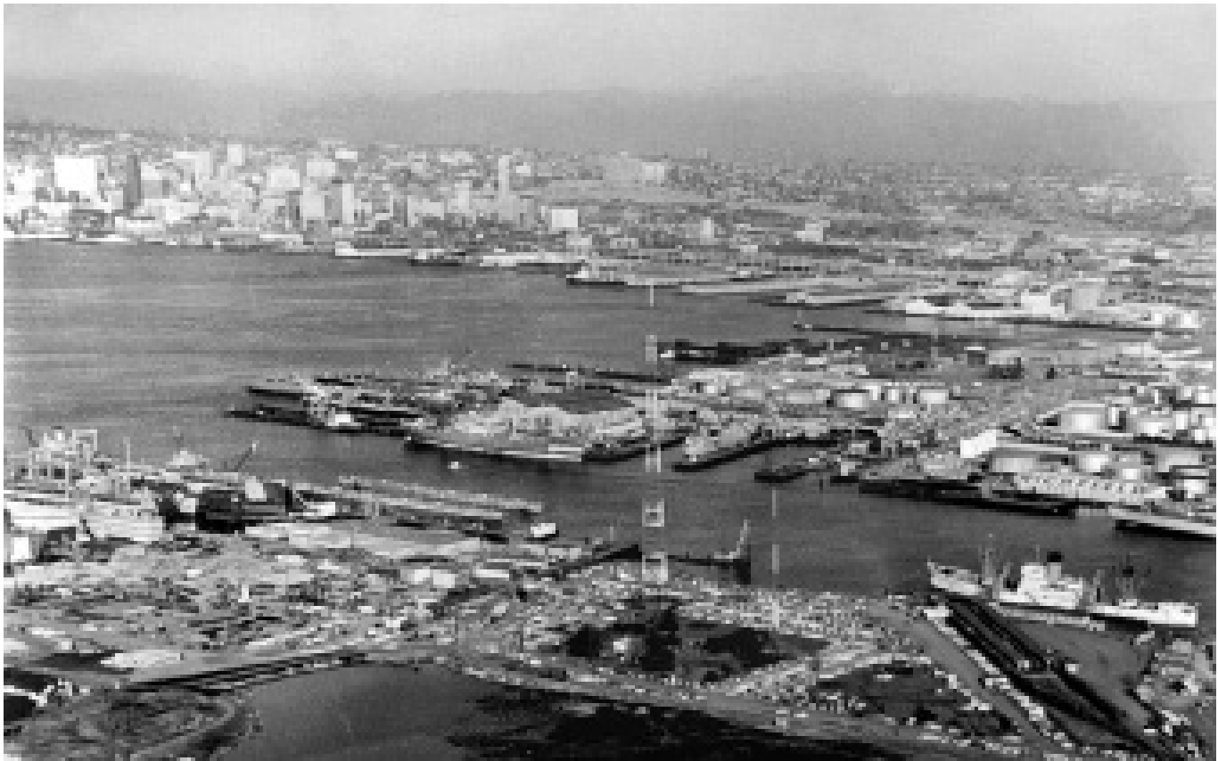
FIGURE 2 | Aerial Views of the KOMO KJR Transmitter on Harbor Island 1964.
