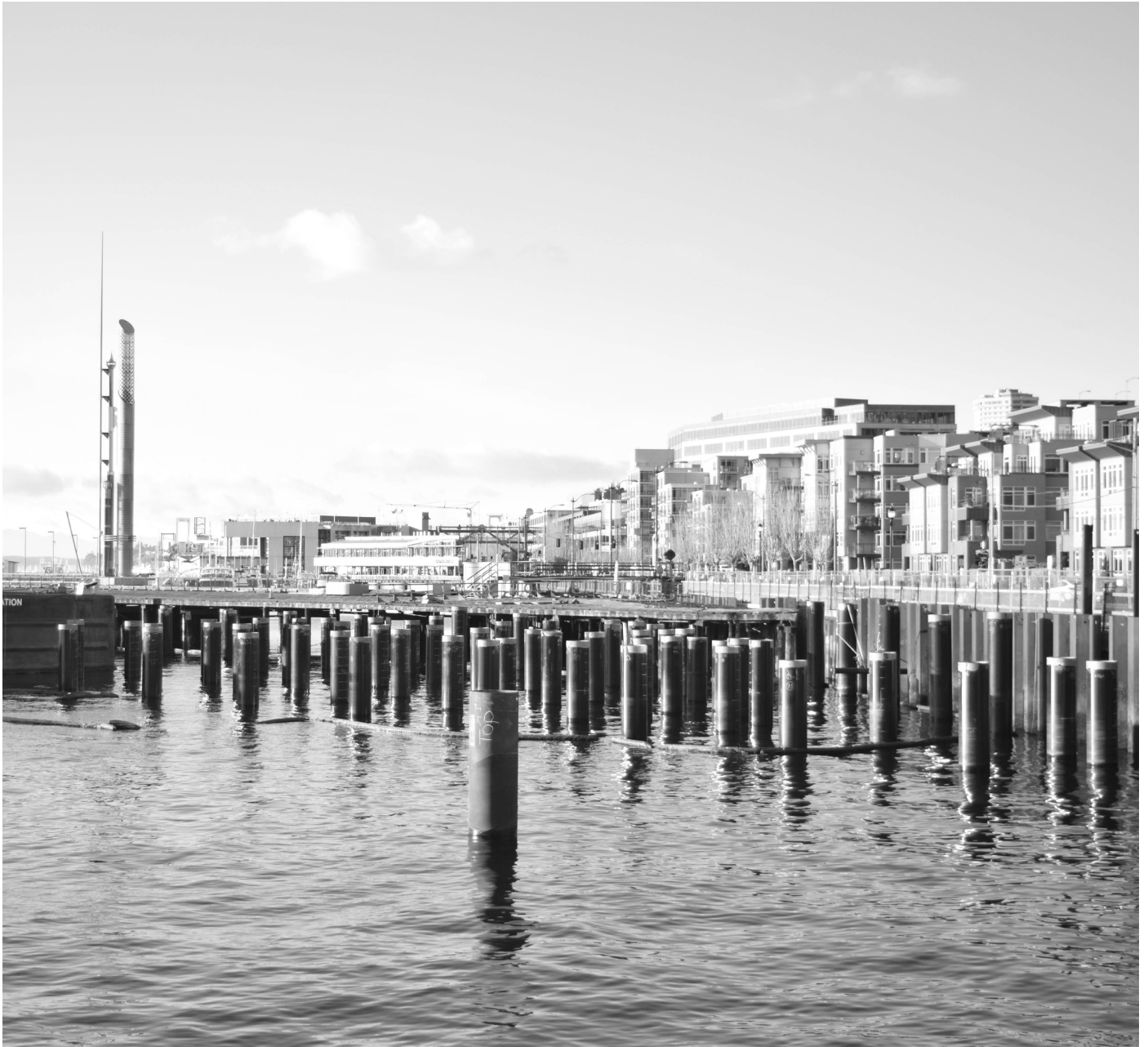
FIGURE 36 | New Pier Construction
