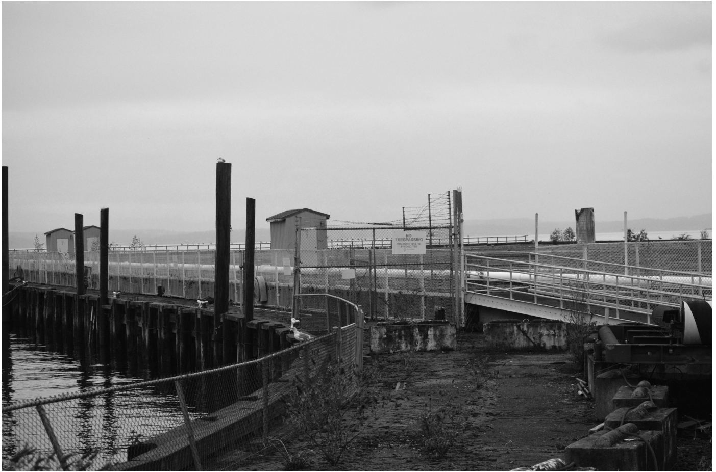
FIGURE 44 | Construction Tied Up At The Site 2
