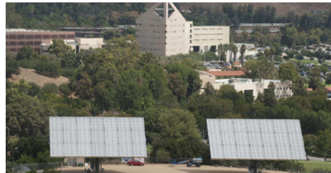
Figure 23- Center Solar Arrays
