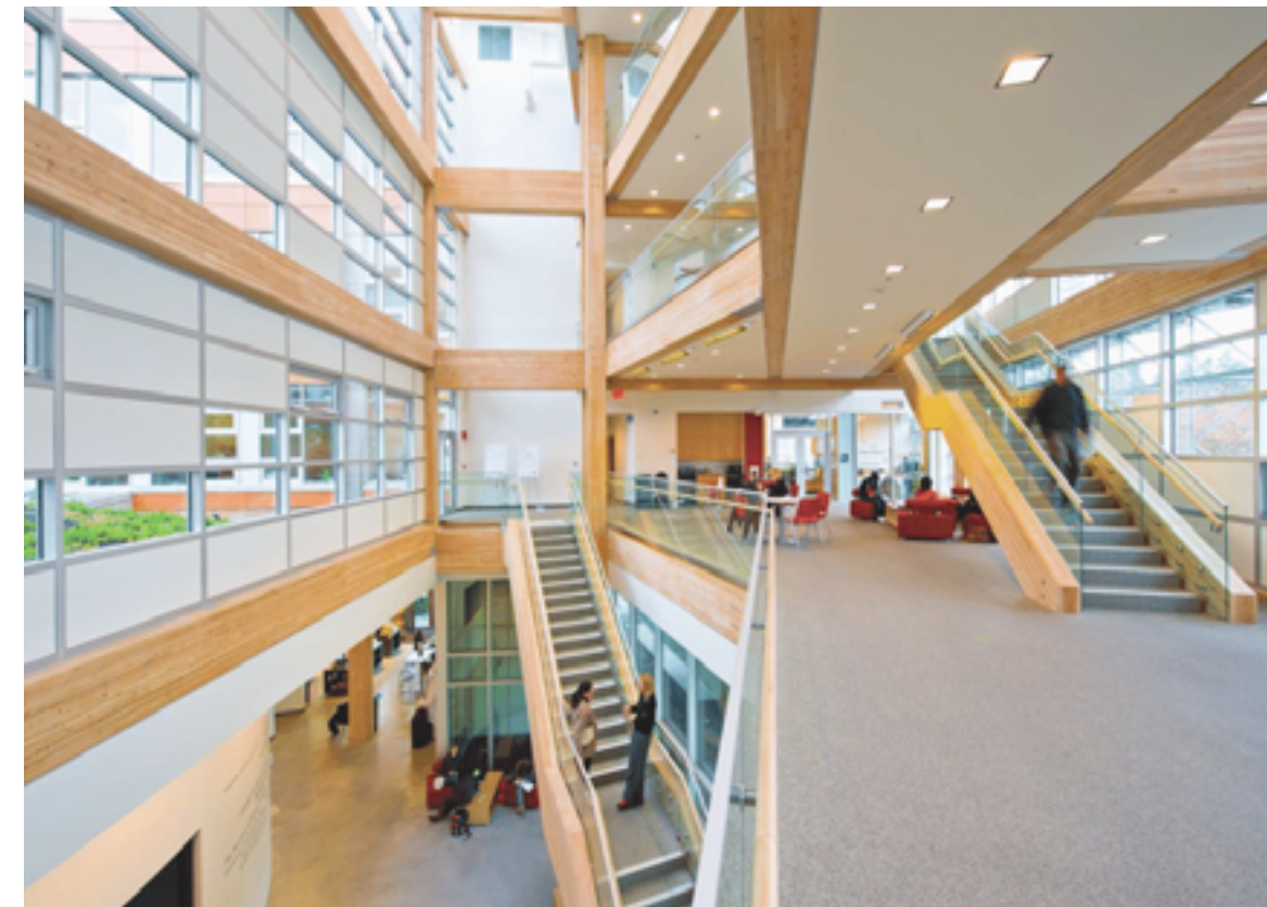
Figure 5. Interior view of the engineered wood members
