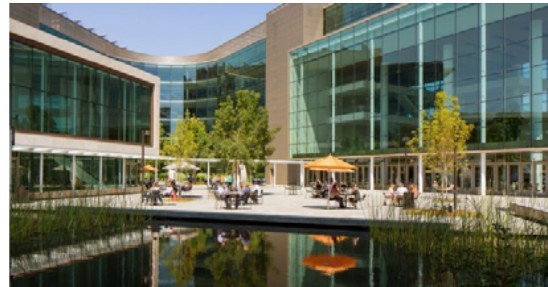
Figure 22- Center Constructed Wetlands
