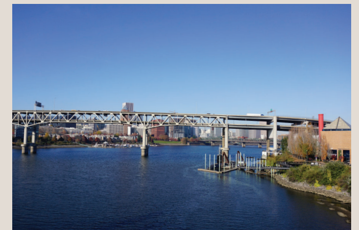
View to the SE of the site looking off Tilikum Crossing
