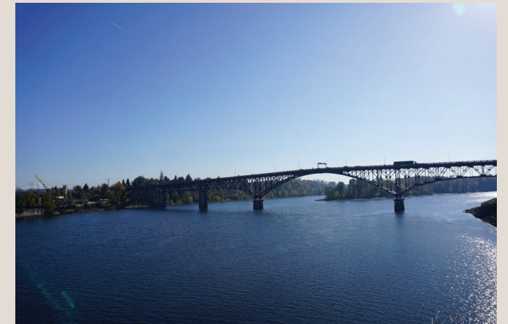
View on Tilikum Crossing to the N of the site
