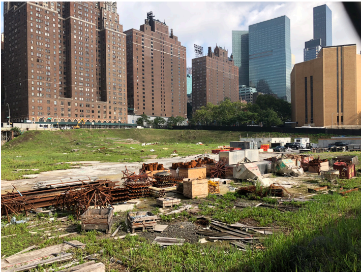
Construction Materials on Site
