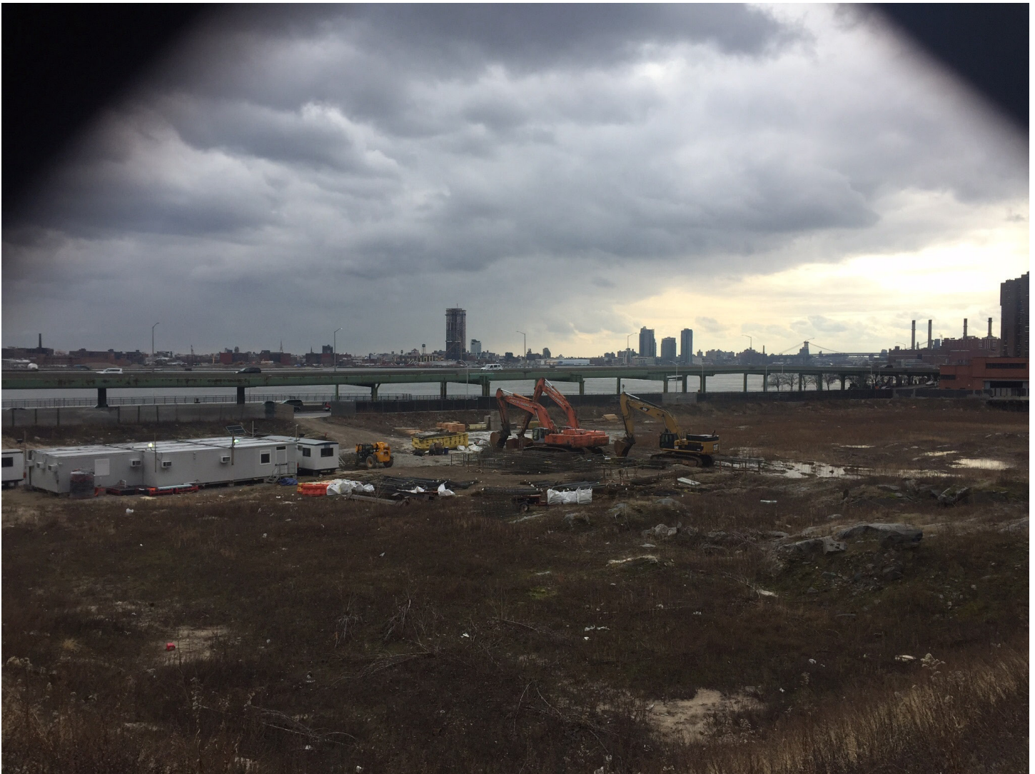
Figure 99: Construction Equipment at the Project Site
