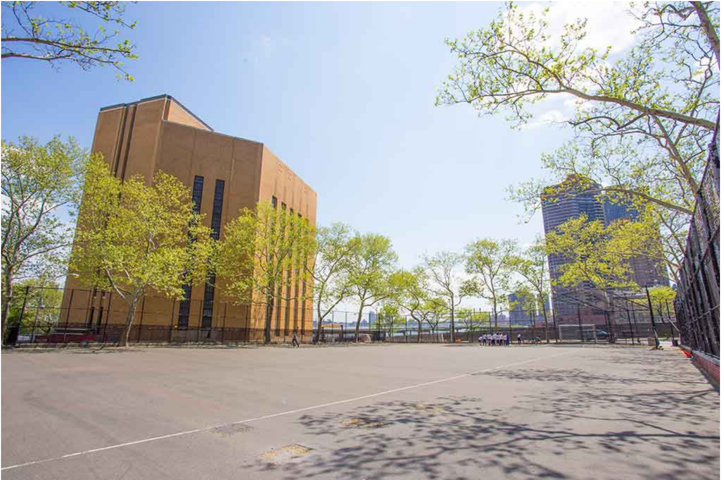
Figure 95: Queens-Midtown Tunnel Ventilation Building
