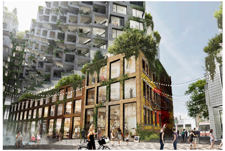
Figure 19: Project Sits on Top of the Preserved Historic Buildings
