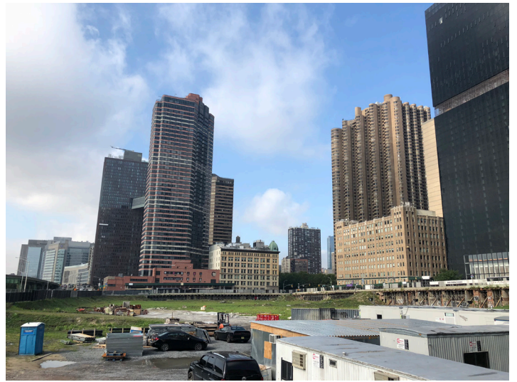
Northeast Corner of Site Facing South
