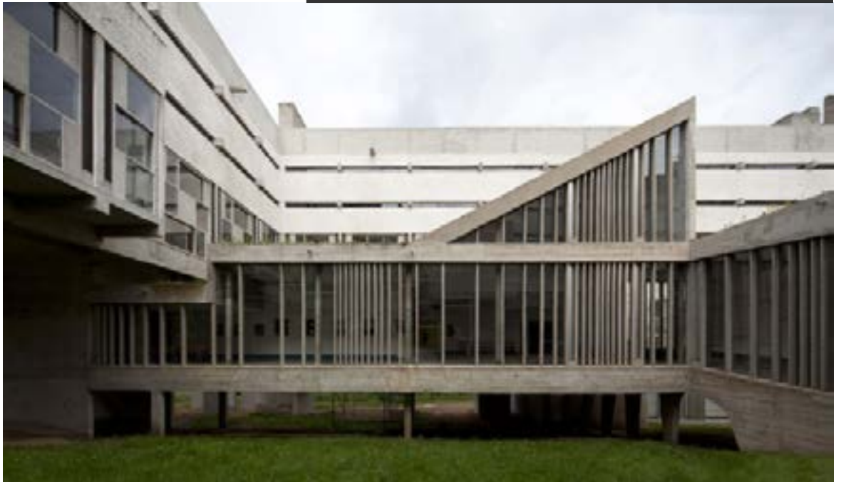
The use of voids in the thick concrete creates a beautiful display of light within the residences as well as giving all residents great views of the landscape that surrounds them.
