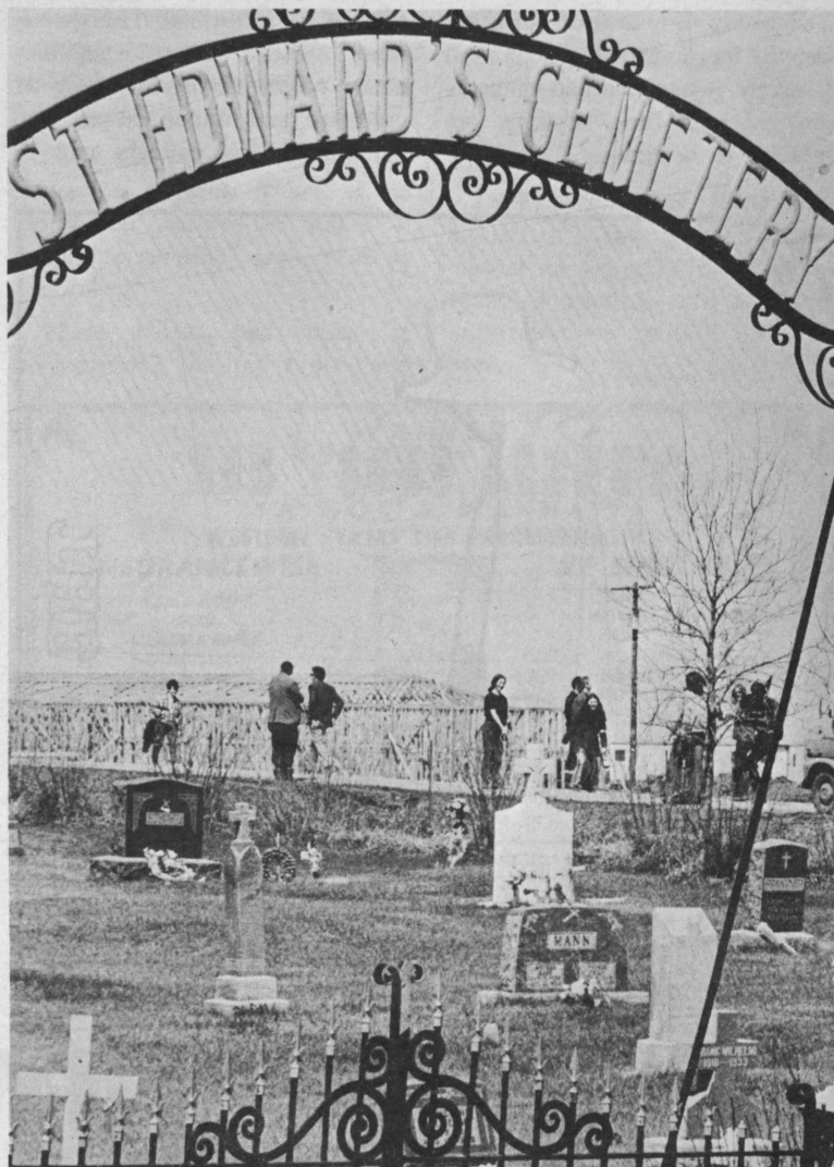
ABM construction buildings lie in the background of a seemingly symbolic cemetery near Nekoma. (Photo by Zielsdorf)
