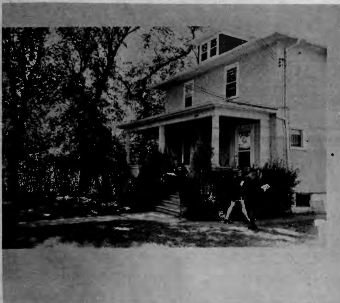
This is the new girl's Co-op house at 1234 11½ St. N. The building was remodelled during the summer and 13 girls are currently living there. The Co-op plans to eventually add more rooms to the house. (See story, page 6)
