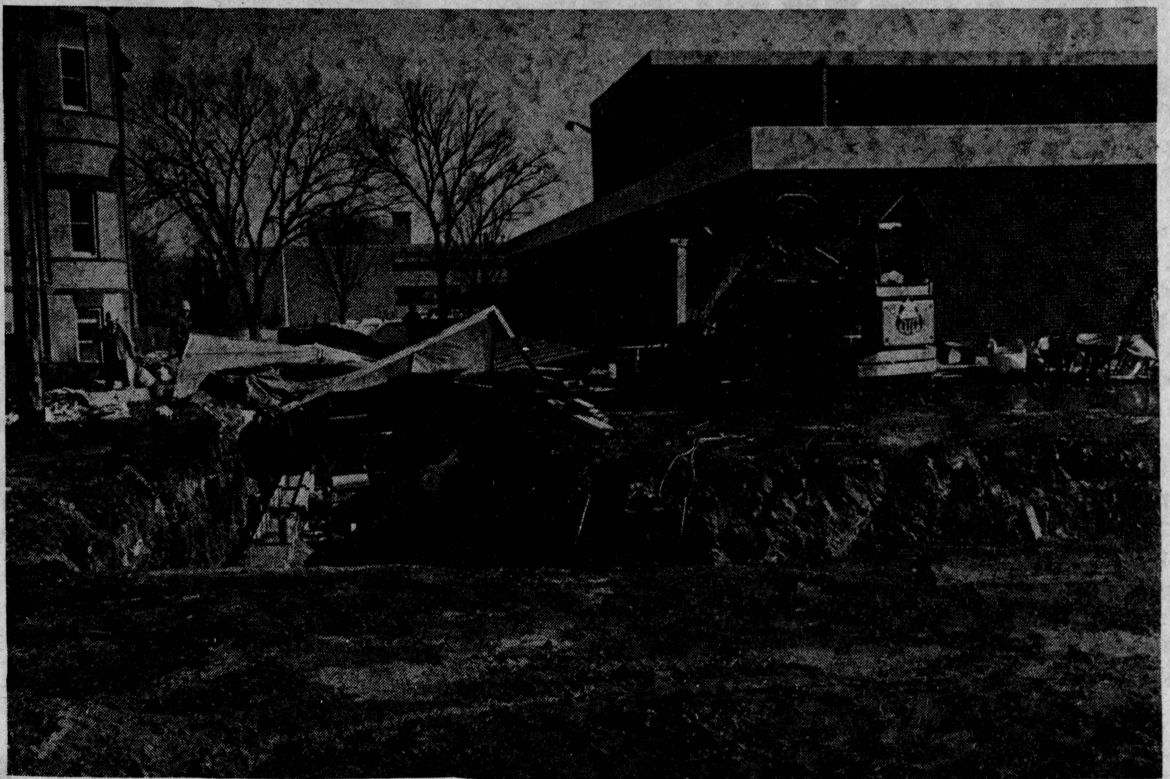
Construction continues on Askanase addition.
