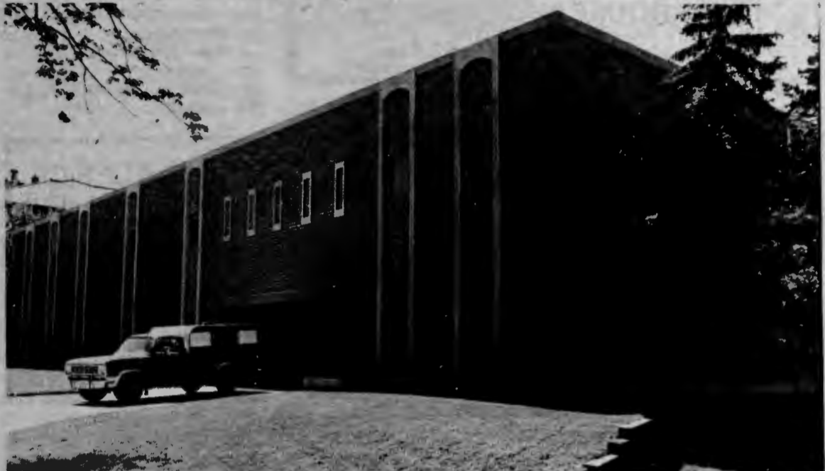
The exterior is now complete on the new Ag-Sci building.
