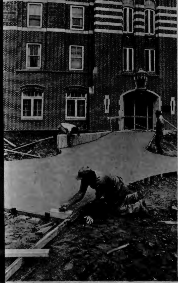
Construction work goes on behind Churchill Hall. (Photo by Grins)
