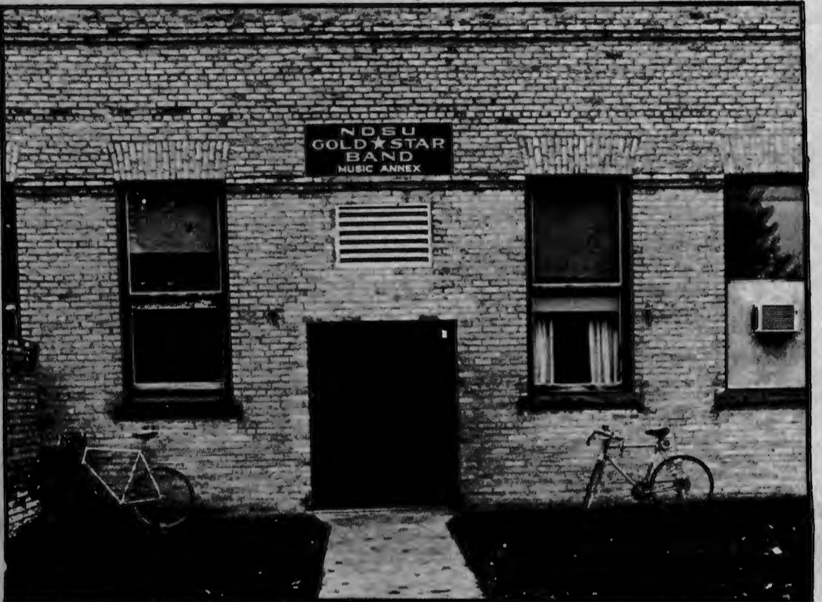
Music classrooms in the South Engineering Annex will soon be housed in a new building. (Photo by Don Pearson)
