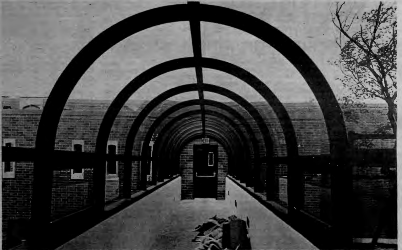
Left: An overhead walkway connects the new Agricultural Science Building to Morrill Hall.
