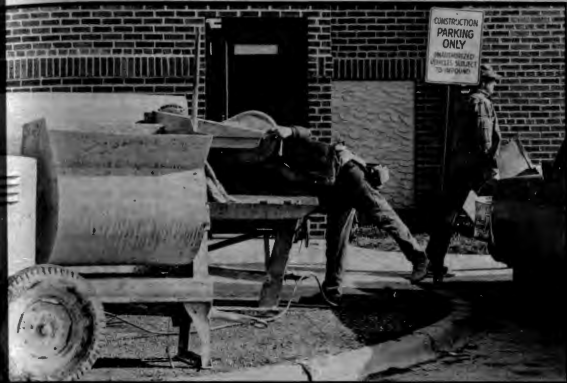
Construction begins on remodeling the Old Fieldhouse
