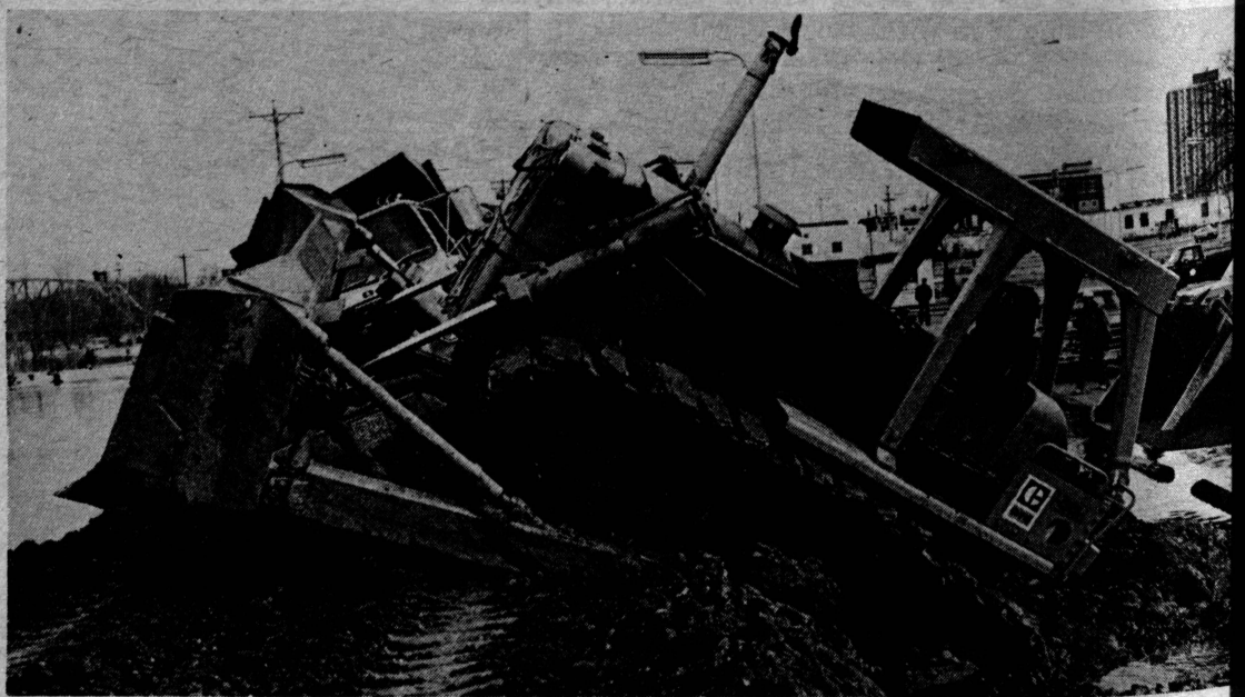
A catapillar works on leveling the dike that was placed on 2nd Street North.
