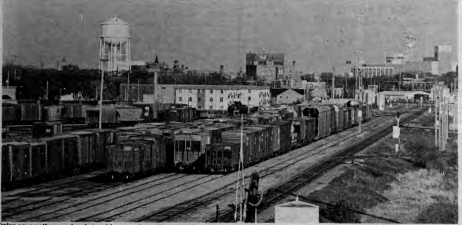
Trains are creating a major obstacle for a number of Fargo residents while the 12th Avenue bridge awaits completion. This shot was taken from the top of the partially completed bridge. There's a story and more photos on page 12. (Photos by Don Pearson)
