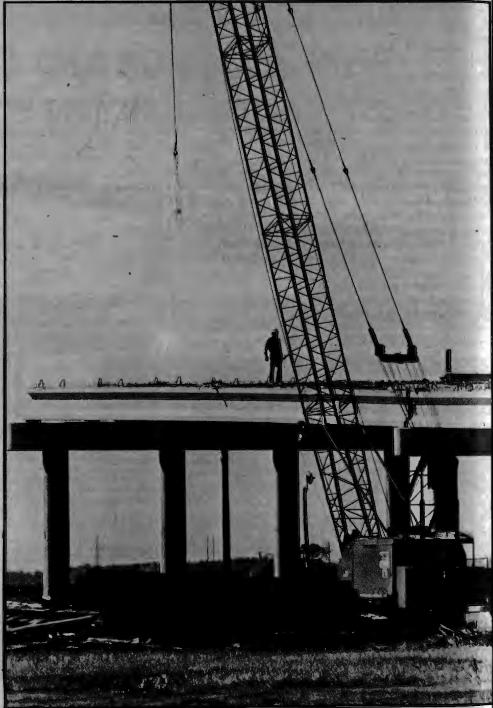
The crane lowers materials to the waiting workmen.
