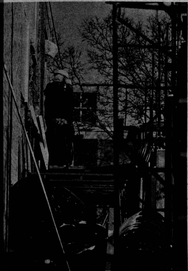
Construction work continues on the addition to the library, here some workers cover up holes in the wall of the old building.
