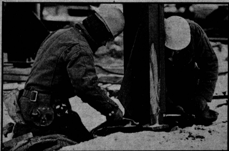
Workers bolt down one of the steel girders.
