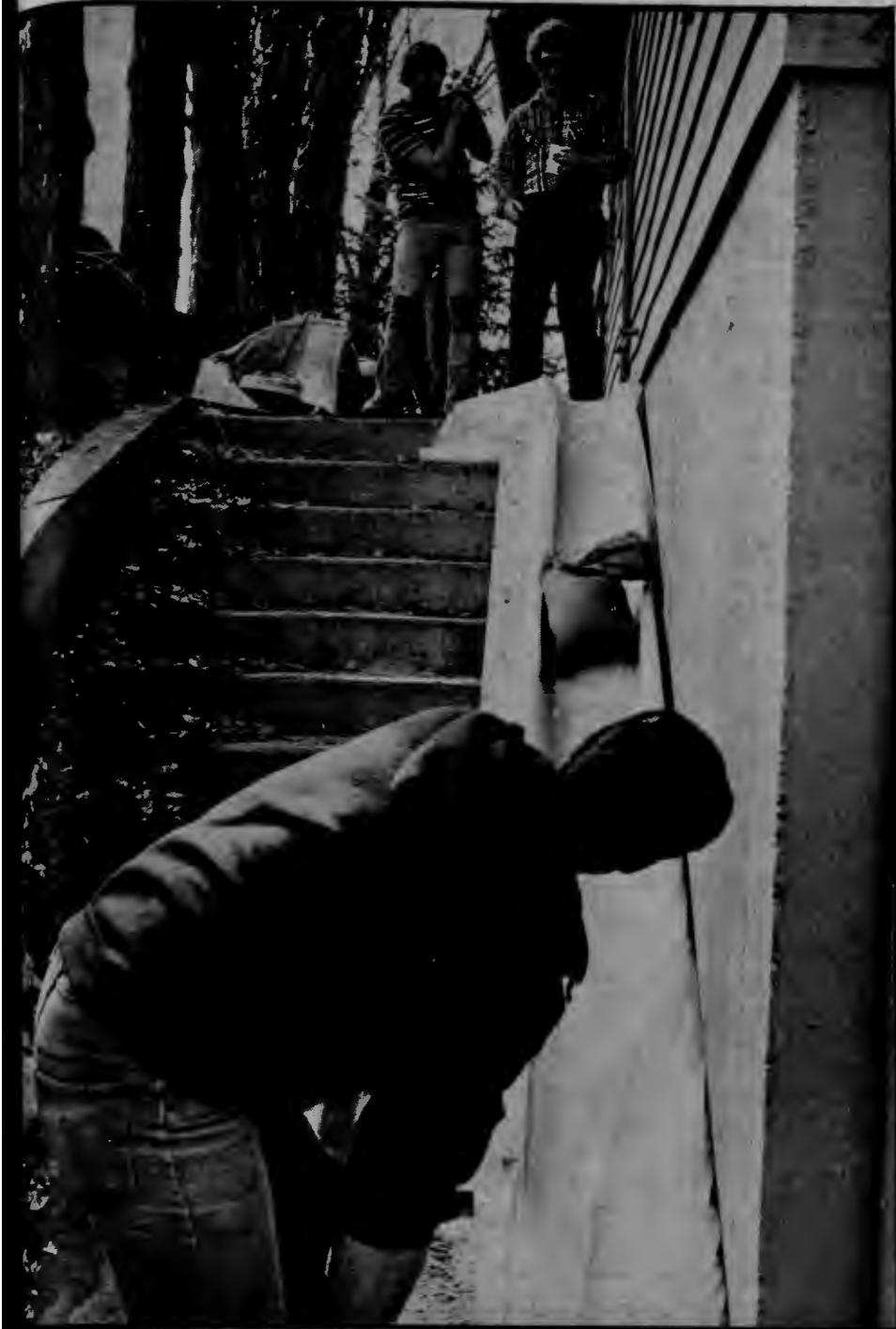
John Peterson and Eric Miller send the sandbags down a slide to a waiting Boyd Zavalney. The slide was used to avoid having to haul the sandbags down the stairs.
