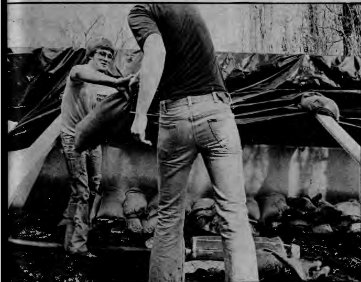
AGRs try to build the wall of sandbags up high enough to hold back the ever rising waters of the Red River.
