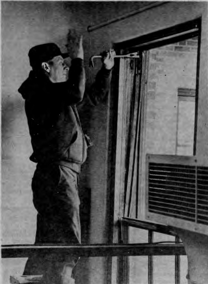
All the old storm windows and the window mounted airconditioners in Morrill Hall are being replaced by new insulated glass and opaque panes. The new windows will be more energy efficient and the new ventilation system will cool the entire building.
