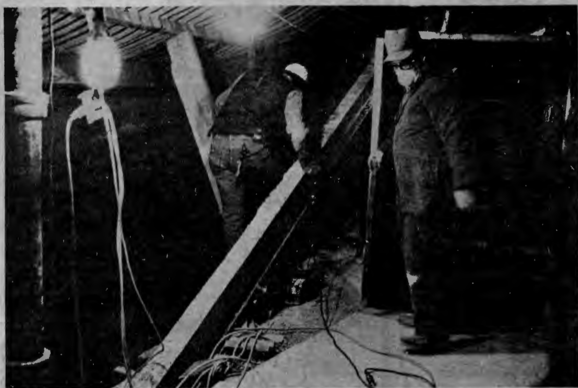
Construction workers are breaking through the walls and floors of Morrill to put in new ventilation system ducting. Eventually, most of the ducting will be covered by false ceilings and new walls.
