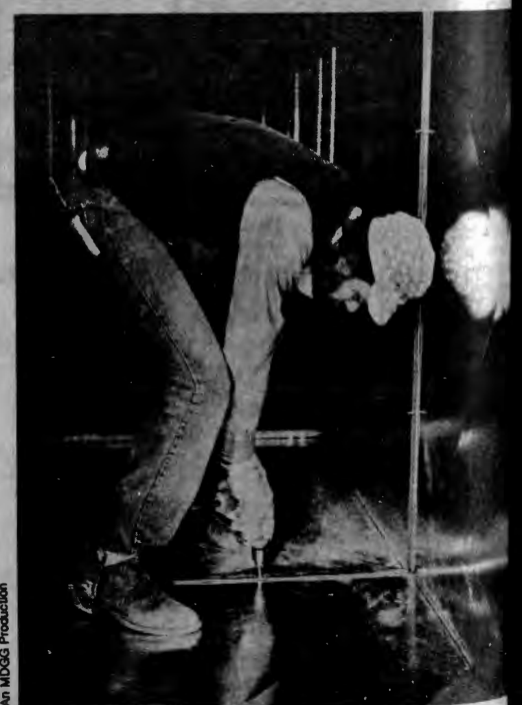
Construction workers are breaking through the walls and floors of Morrill to put in new ventilation system ducting. Eventually, most of the ducting will be covered by false ceilings and new walls.
