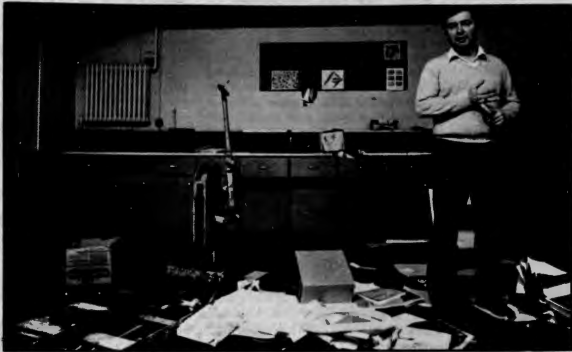
(Above and below) Agricultural Communications department head Dr. Chuck Humphrey lists the improvements to be made to Morrill Hall in the next few months.
