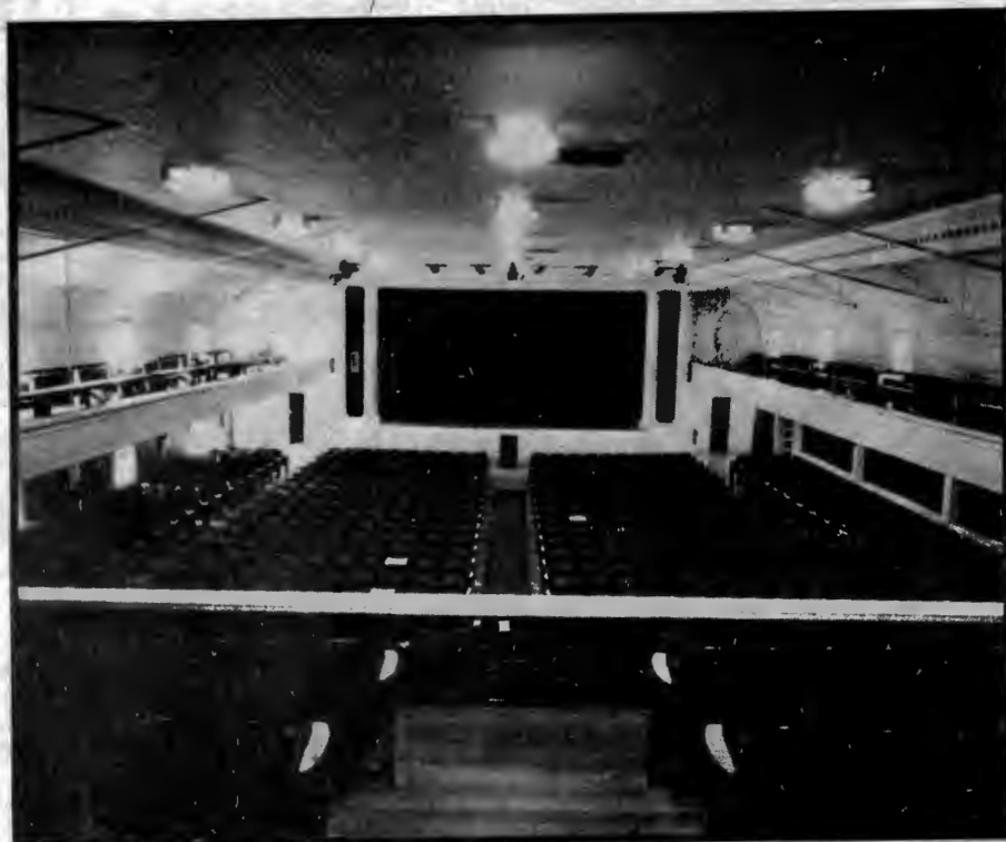
Festival Hall from the inside looks gloomy before demolition begins.
