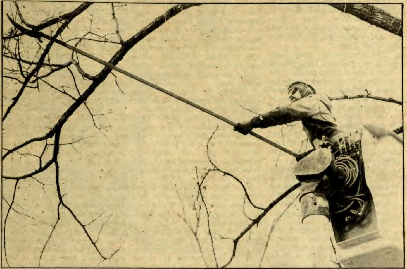
Danny Glaser of 801 28th St. N. in Fargo stretched to trim a branch with a long-handled saw. This type of saw is necessary to reach branches inaccessible to the basket because of electrical wires.
