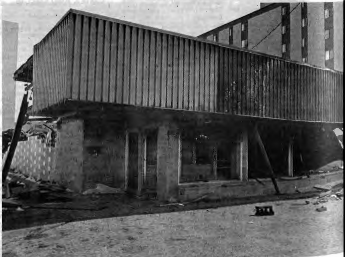
The remains of the old ARC thrift store at 215 North University that was gutted by fire on Feb. 9.
