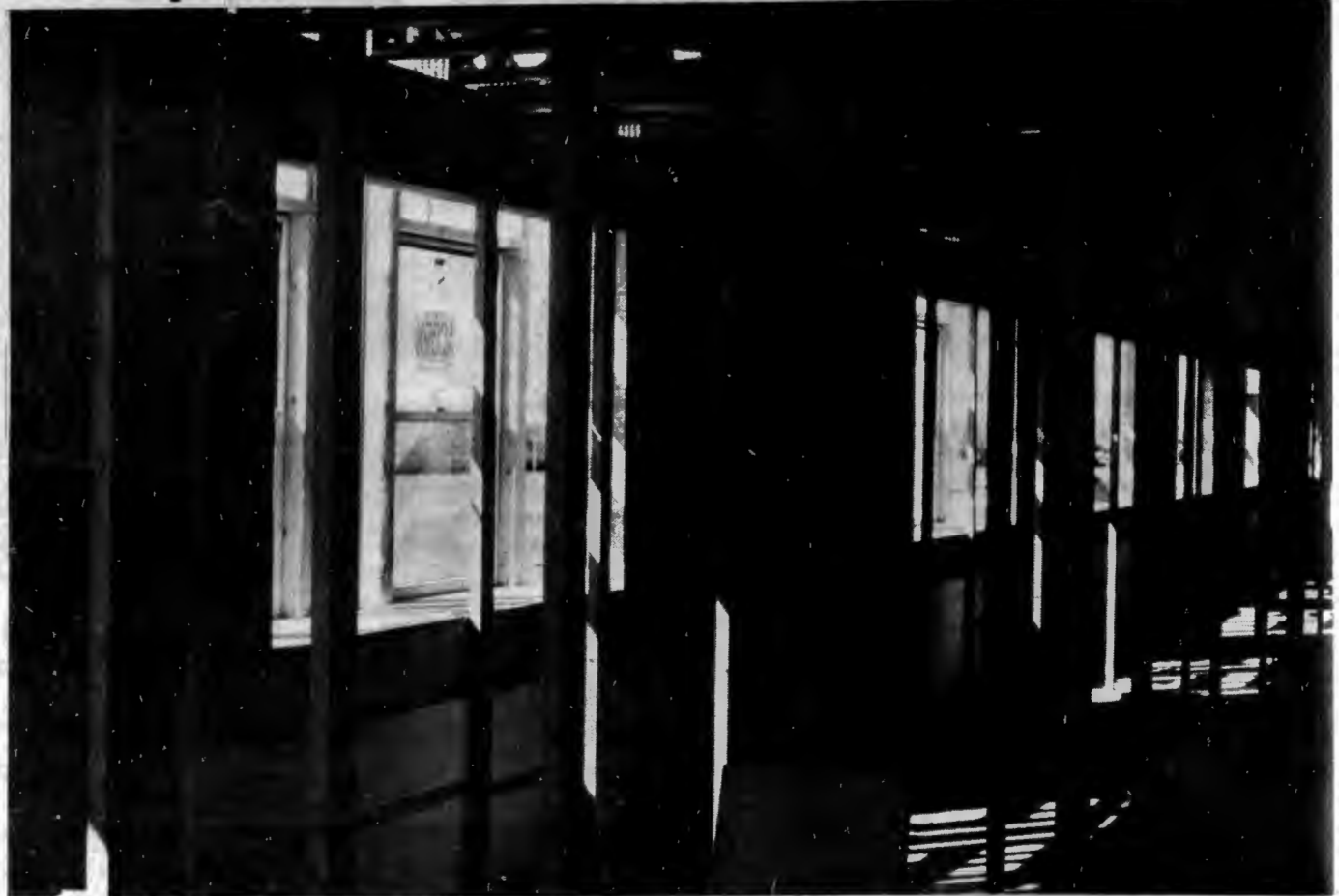
It's dark and spooky now, but this new 16-unit apartment building should be housing students by the end of fall quarter. (Photo by Kirk Kleinschmidt)
