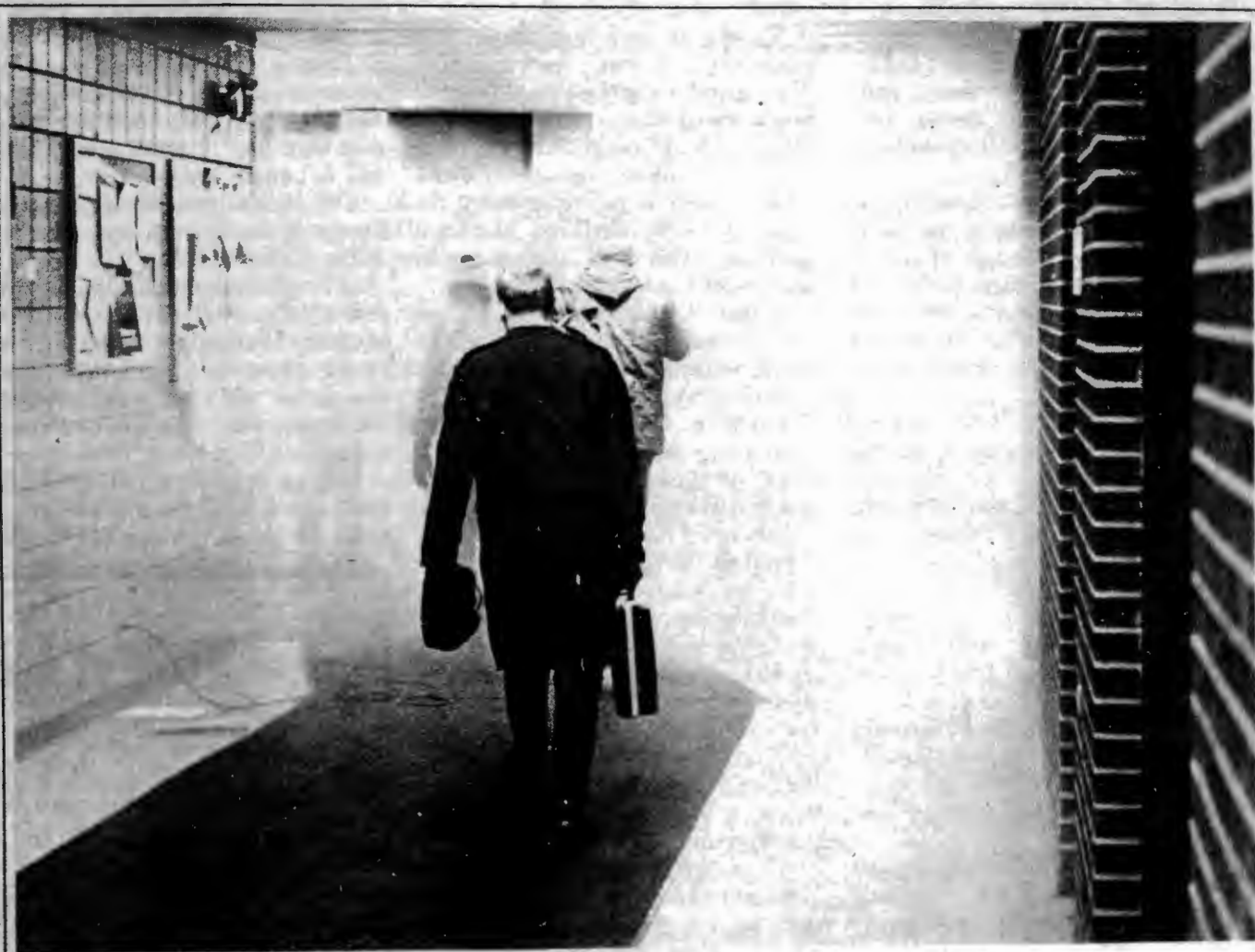
The bursting of a frozen water pipe steams things up for engineering students. (Photo by Jeff Wisnewski)
