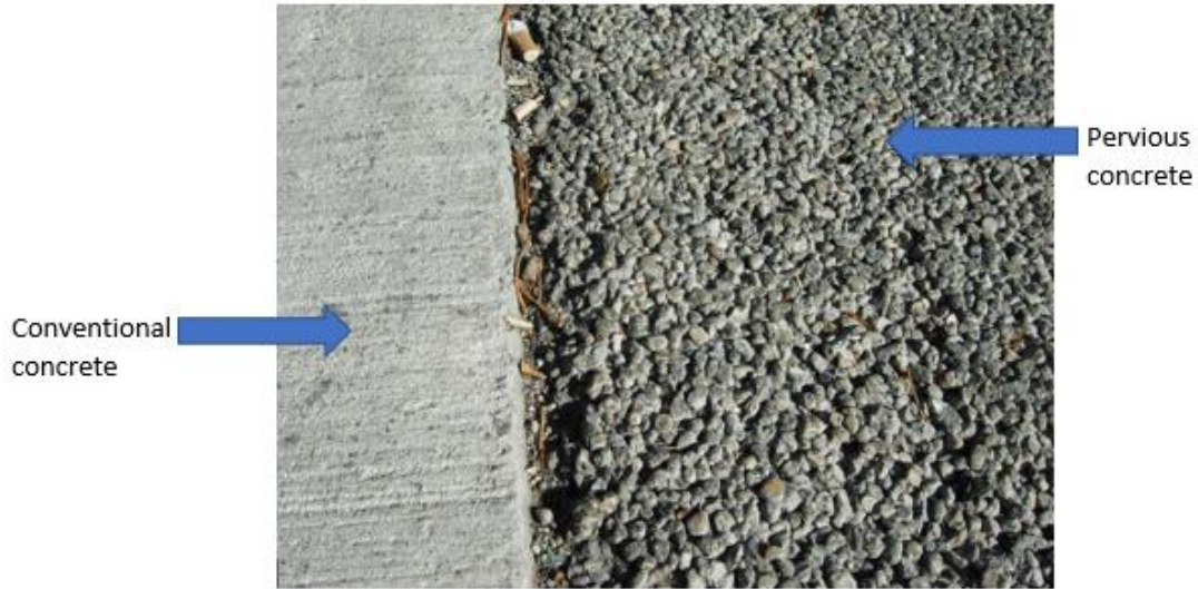
Fig. 1.1. Side by side visual comparison of conventional and pervious concrete [Source: go-gba.org]
