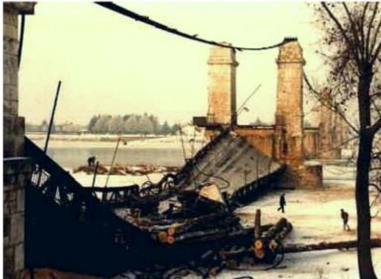
Figure 1. Bridge collapse in France (1986) due to a traffic accident [3]
