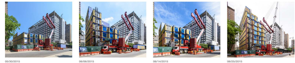
FIGURE 22 | CARMEL PLACE CONSTRUCTION PHASES | HTTP://NARCHITECTS.COM/WORK/CARMEL-PLACE/
