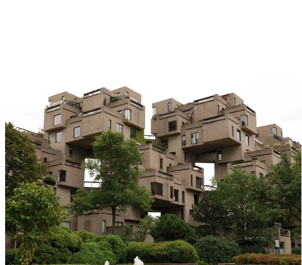
FIGURE 34 | HABITAT 67 VIEW A | HTTPS://WWW.ARCHDAILY.COM/404803/AD-CLASSICS-HABITAT-67-MOSHE-SAFDIE
