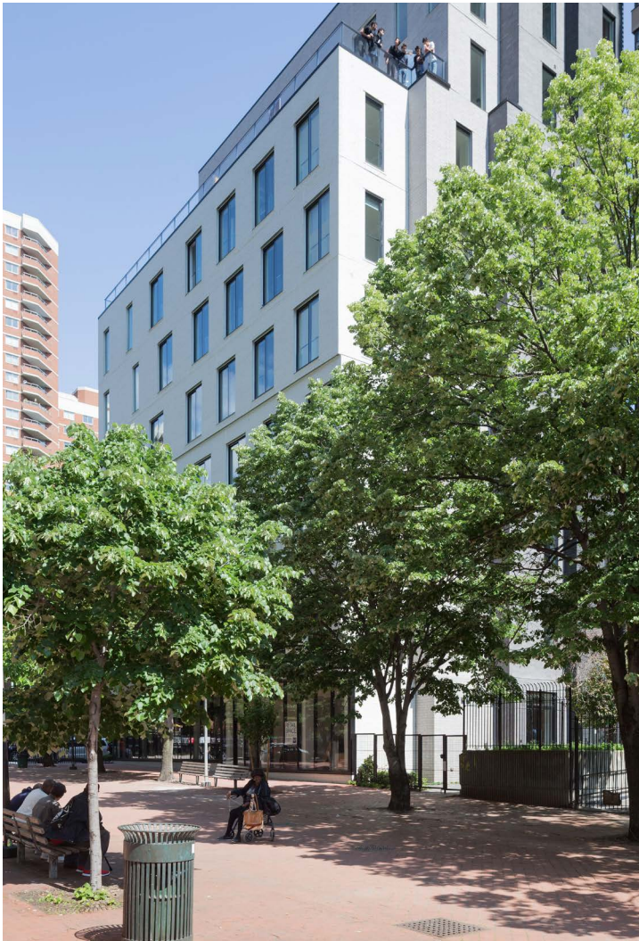
FIGURE 12 | CARMEL PLACE STREET VIEW | HTTP://NARCHITECTS.COM/WORK/CARMEL-PLACE/
