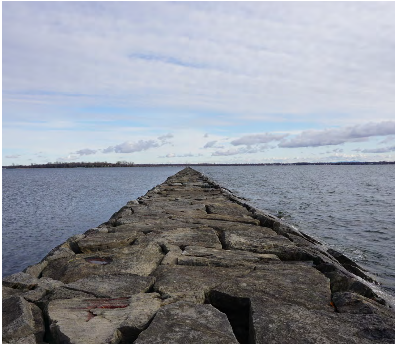
Figure 64 | Stony Point Break Wall - Photogrid B
