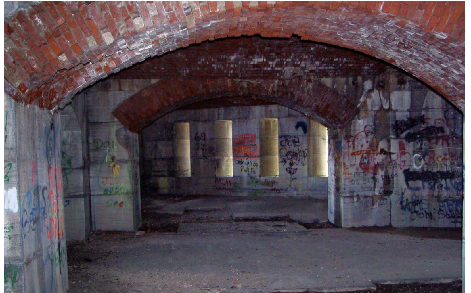
Figure 83 | Bastion C Tier 2 Loopholes - Photogrid U | Jim Millard
