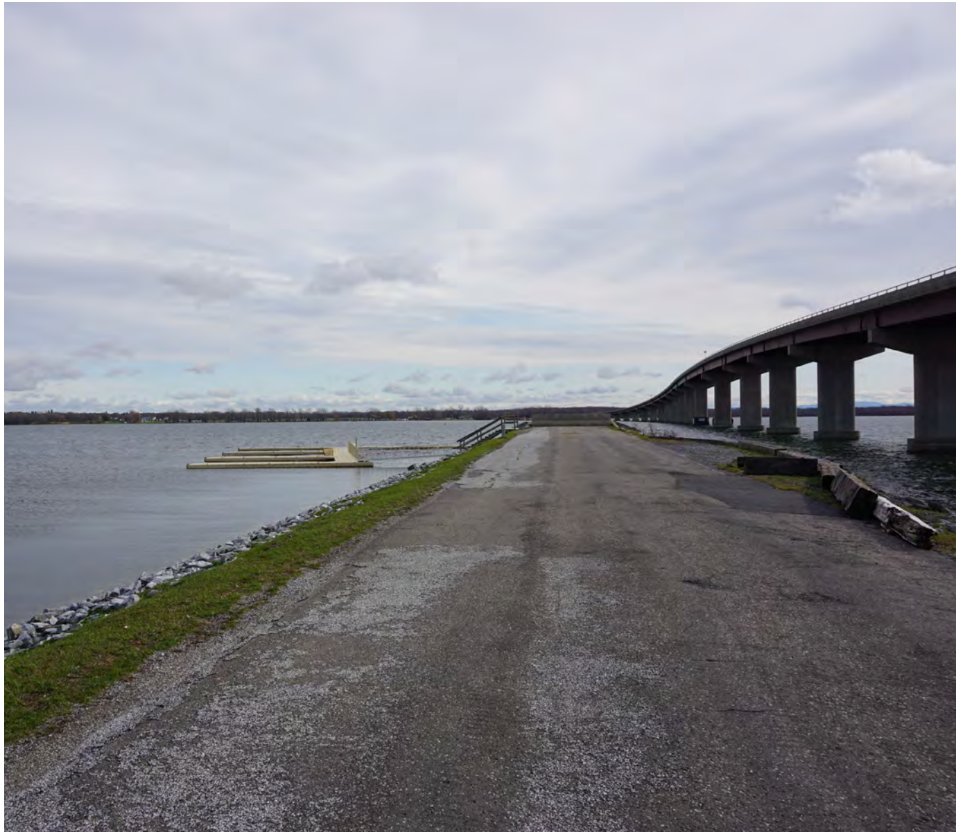
Figure 74 | Frontage Road - Photogrid L
