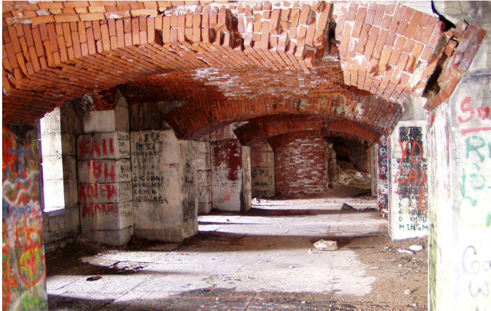
Figure 81 | Bastion C Tier 1 Interior - Photogrid S | Jim Millard
